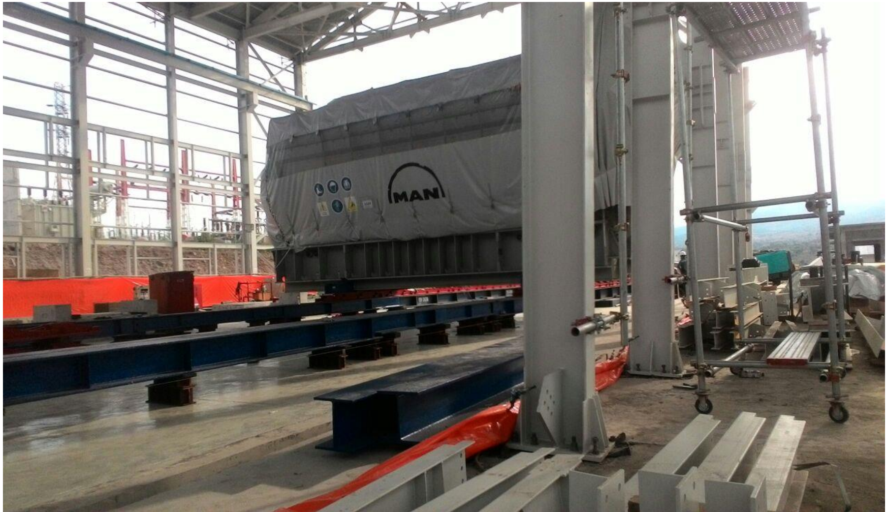
GAS ENGINE ALMOST ON FOUNDATION
