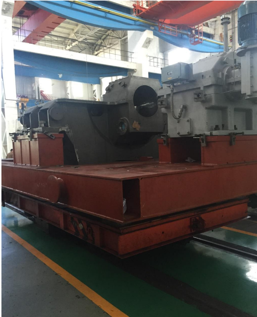
Install Steam Turbine unit
