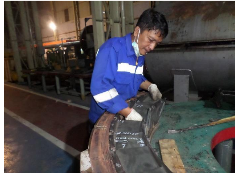
Disassembly Nozzle Segment from Retaining Ring 1st stage Nozzle GE Gas Turbine MS 5002
