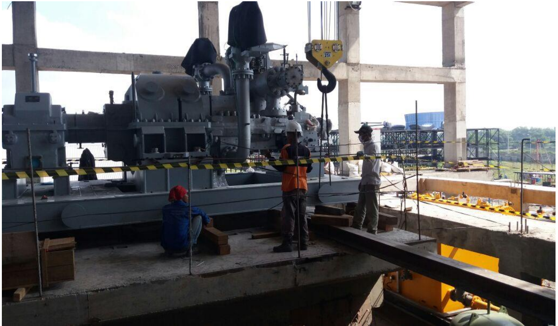
Turbine on position
