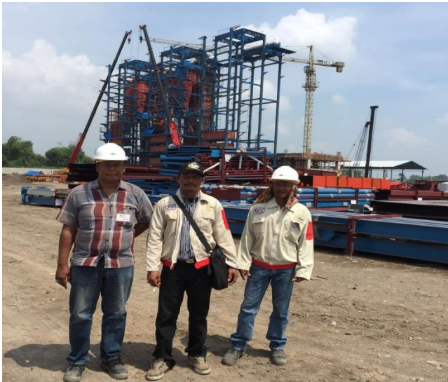
CFB under construction
