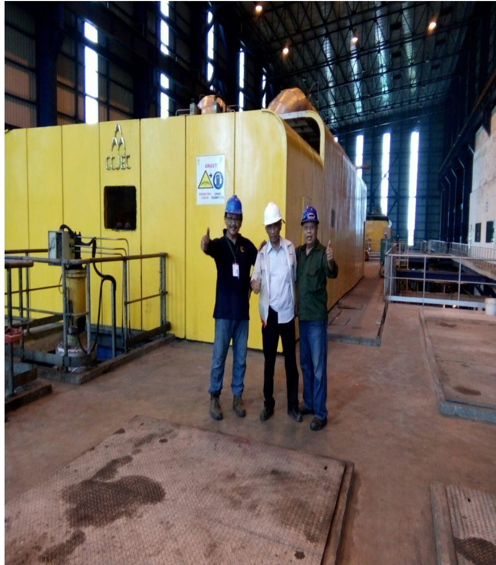
Re-install turbine 100 % completed
