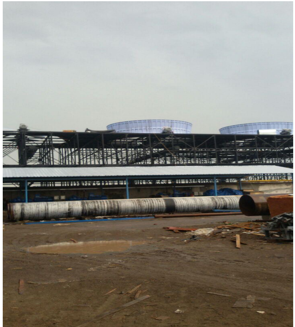
Install cooler tower / cooling water system
