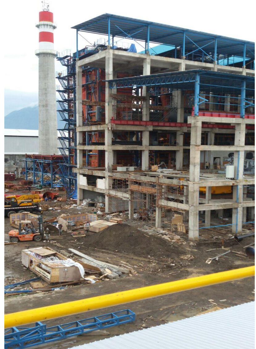
Install electrical / control cable
