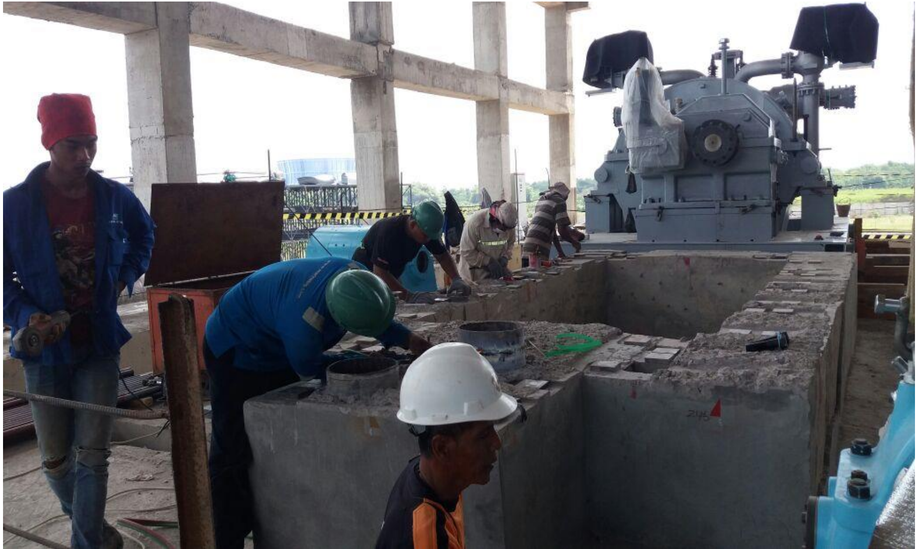
Preparation for lifting Generator
