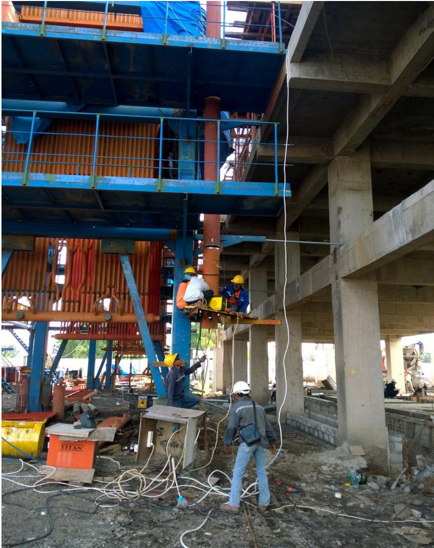
Fit up pipe lower down comer
