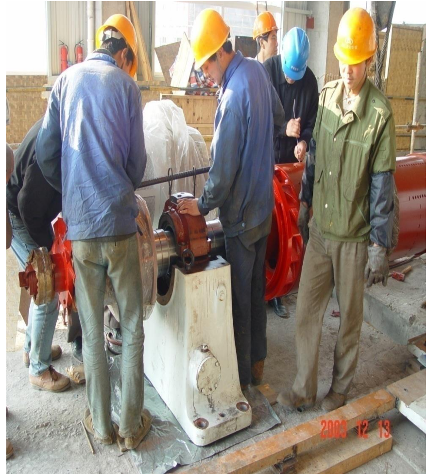
Install Stator and rotor generator unit
