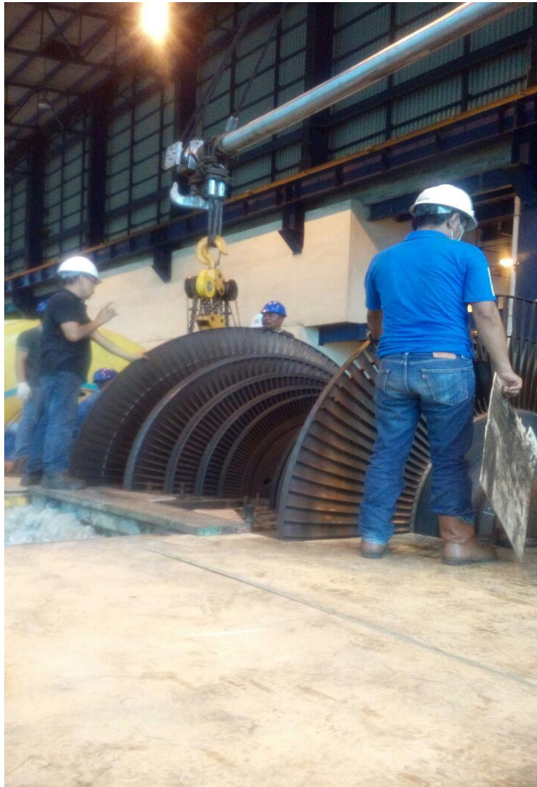
INSPECTION OF LP TURBINE ROTOR
