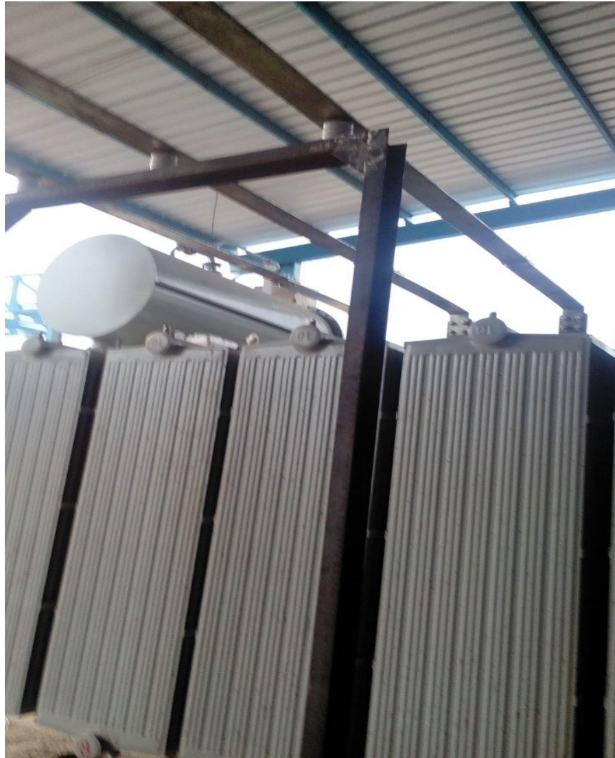
Installation of bush bar
