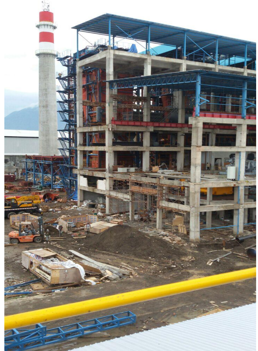
Install overhead crane
