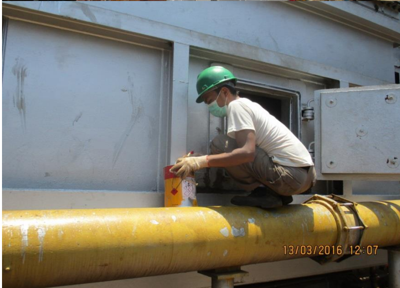
Clean Up and Painting of Exhaust Plenum with Heat Resistance paint
