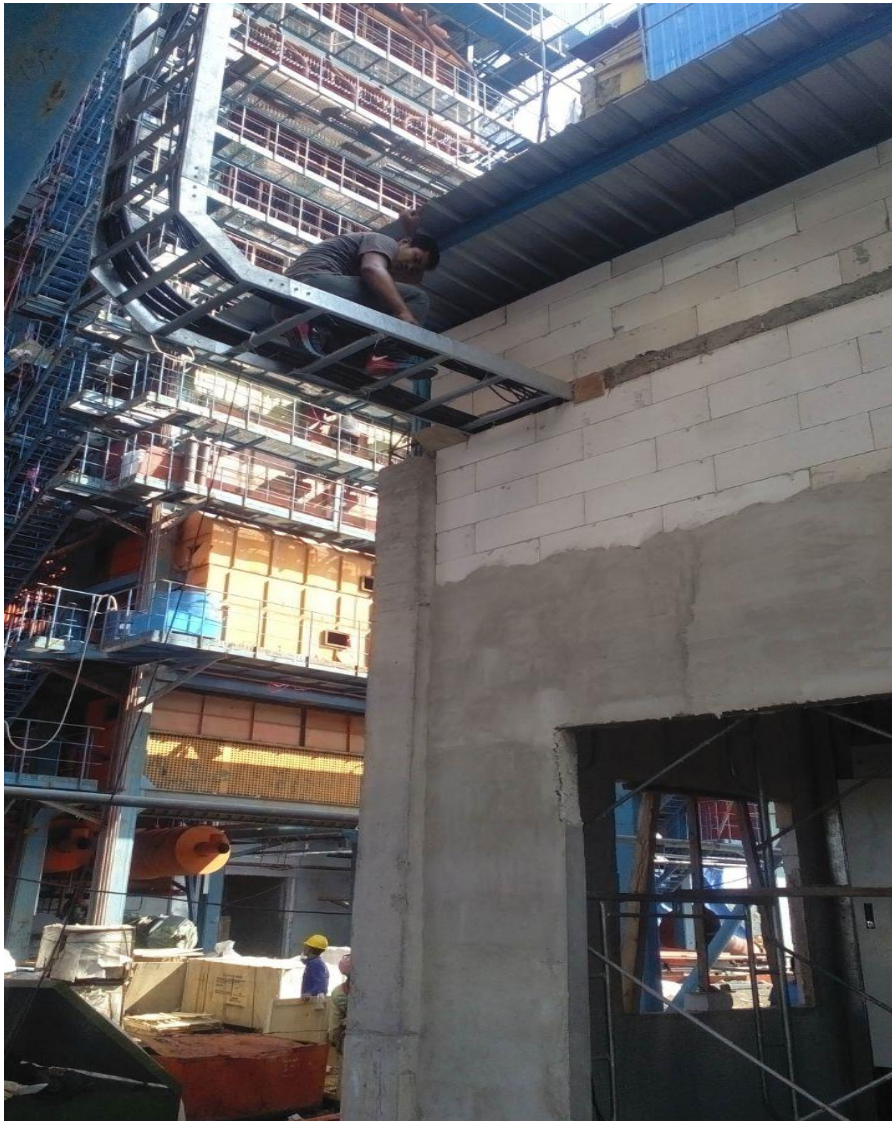
Install electrical / control cable
