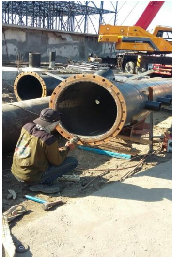
Welding underground pipe
