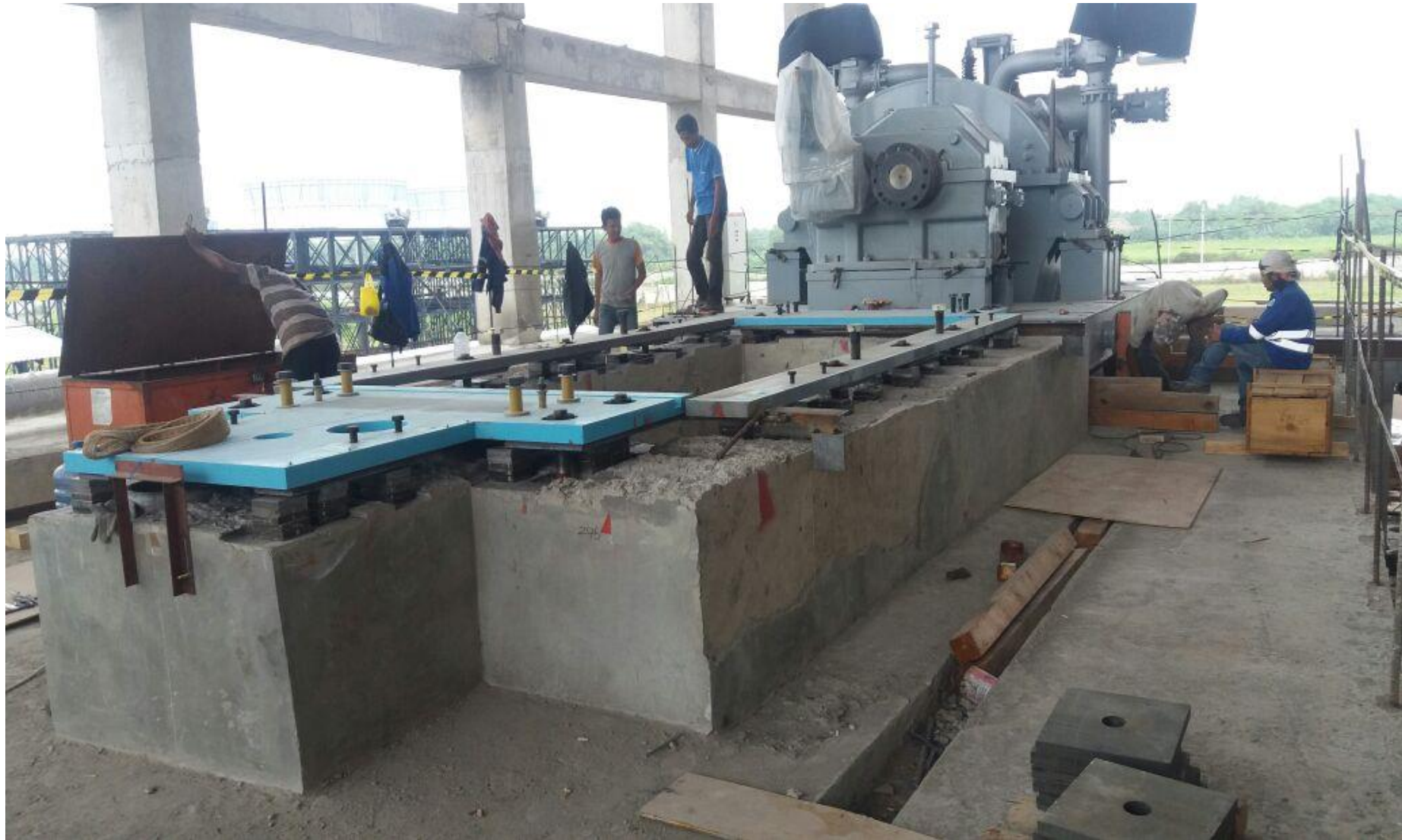
Preparation for lifting Generator
