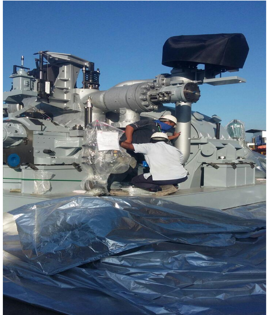
Turbine on position
