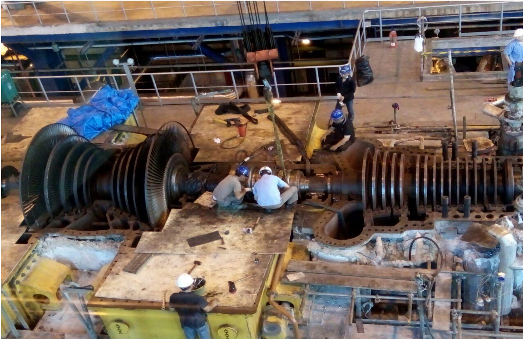
ALIGNMENT HP AND LP TURBINE 110 MW AT PLN SEBALANG LAMPUNG
