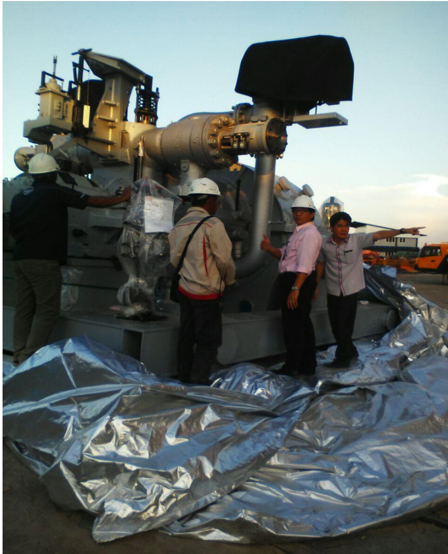
Preparation for lifting Steam Turbine
