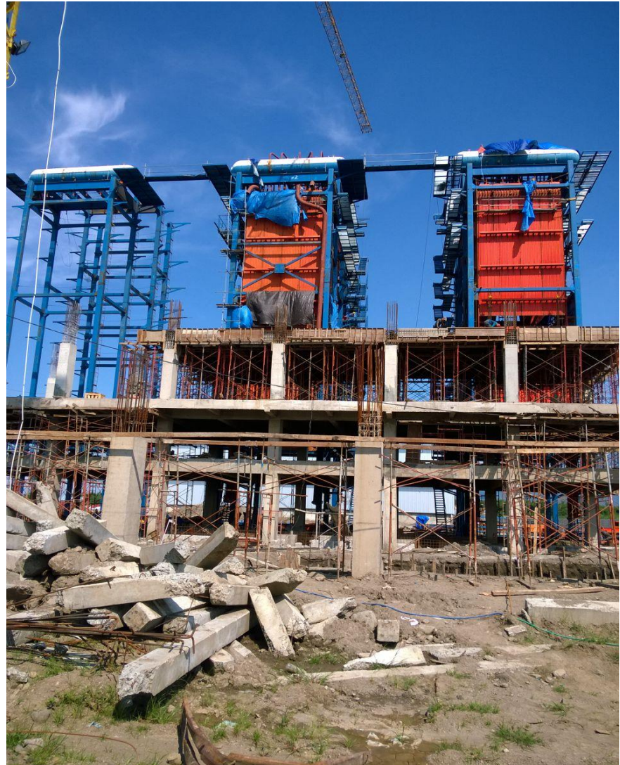
3 ( three ) unit steam drum fix at place)
