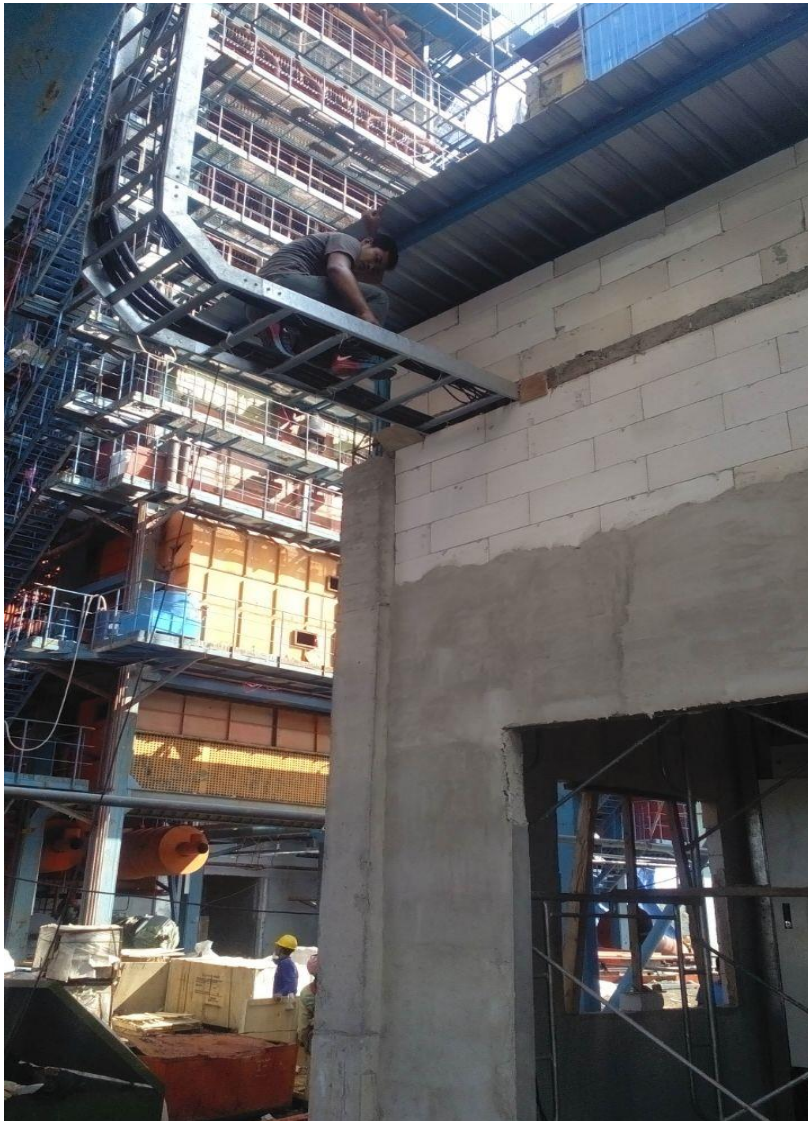
Install electrical / control cable
