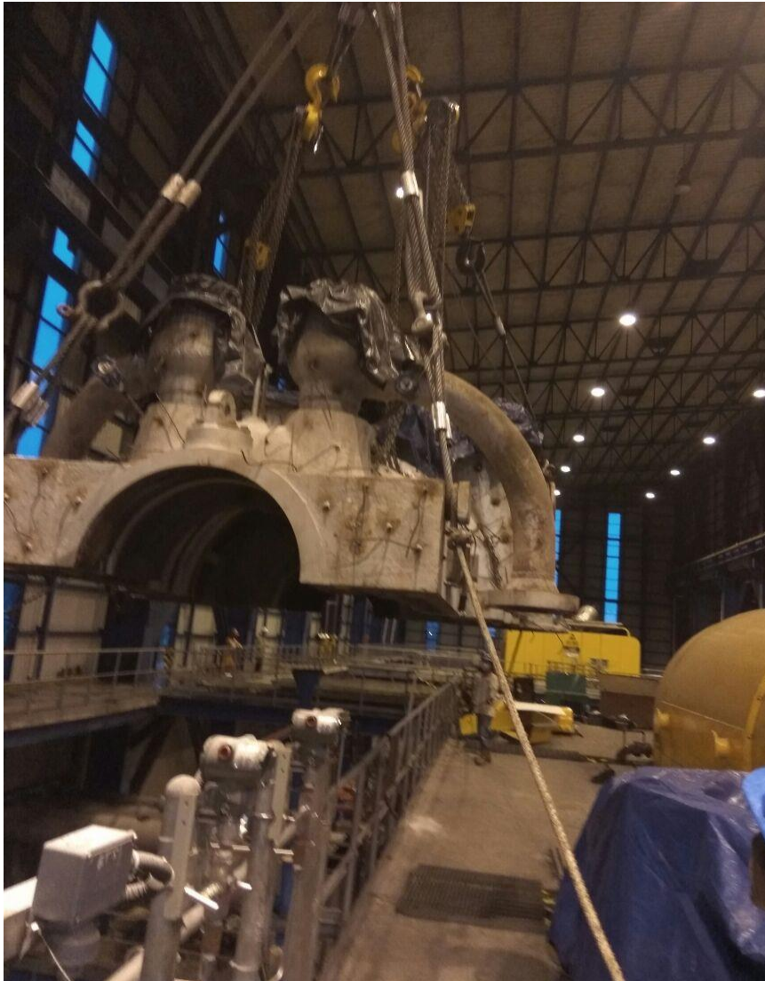
Lifting UPER CASING HP TURBINE 110 MW AT PLN SEBALANG LAMPUNG
