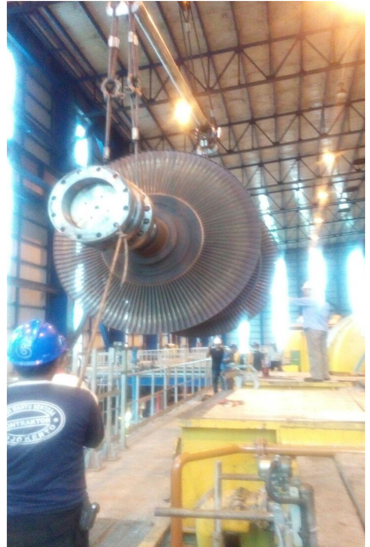
Lifting UPER CASING HP TURBINE 110 MW AT PLN SEBALANG LAMPUNG
