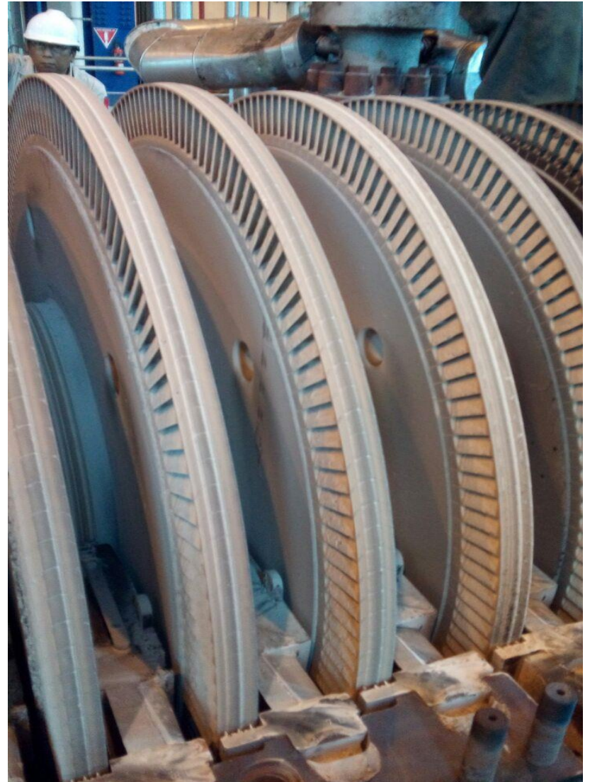
Re-install HP Rotor turbine 110 MW
