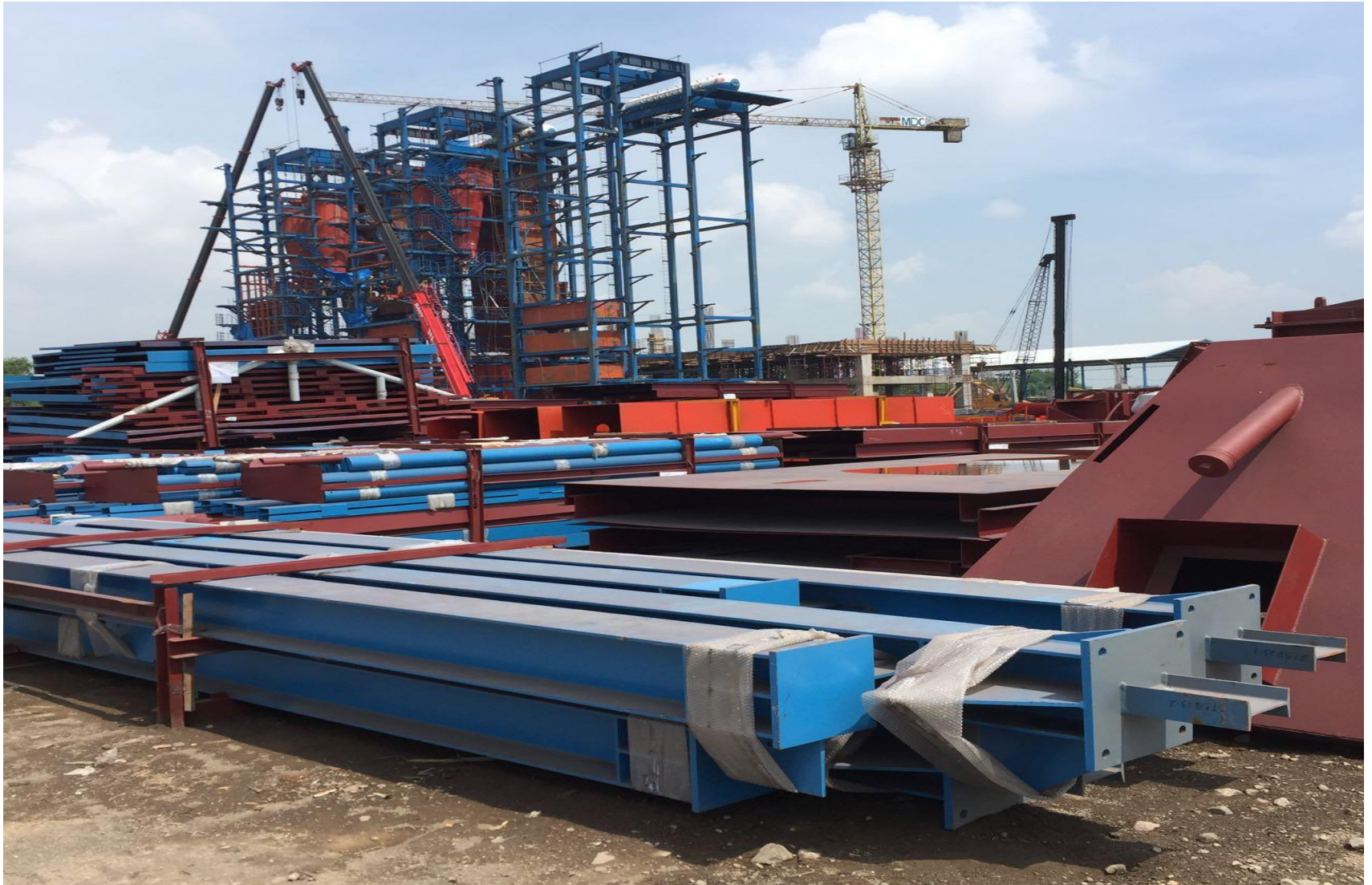
CONSTRUCTION of Steam Power Plant 2 x15 MW at PT. SINERGY POWER SOURCE MOJOKERTO
