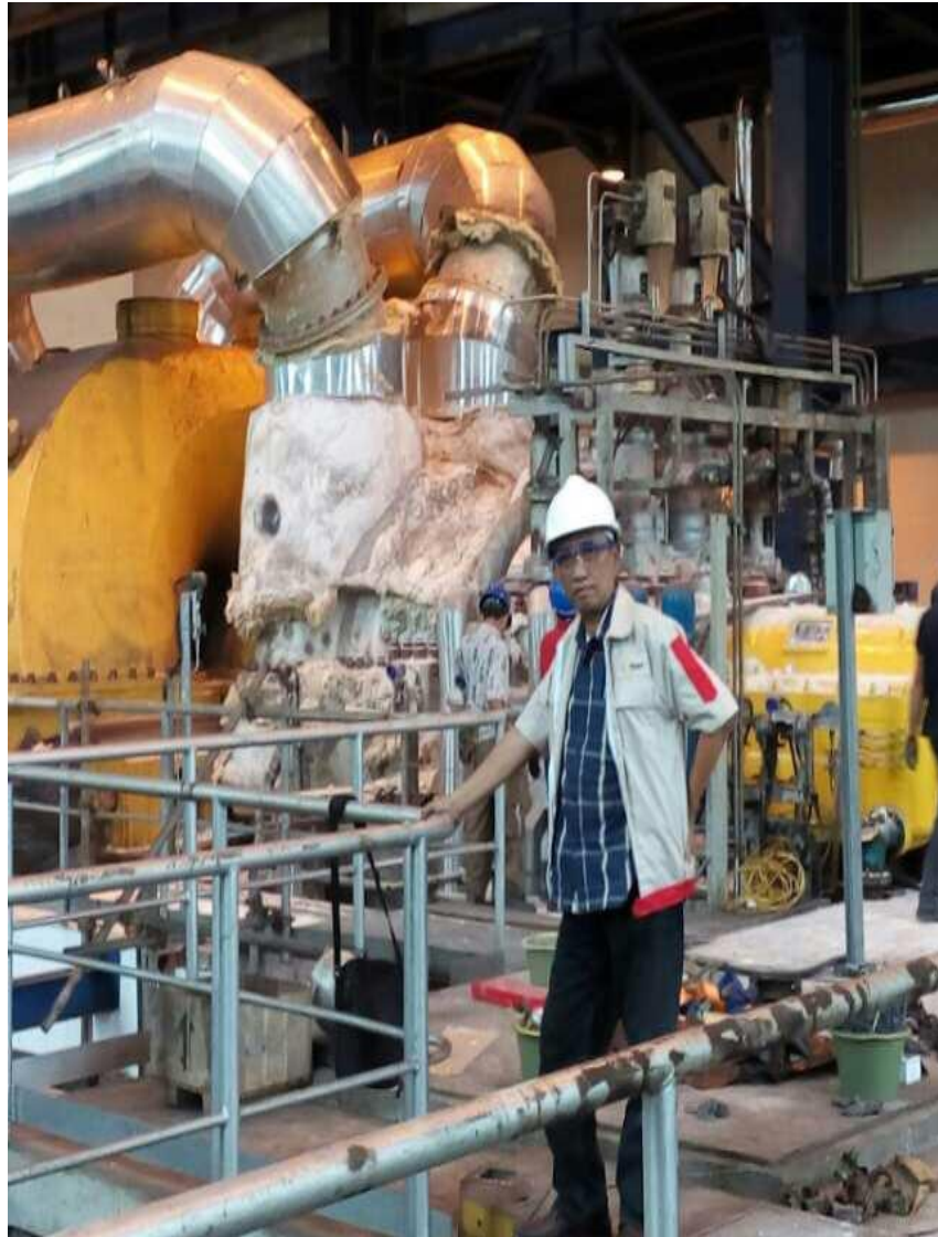
Re-install turbine 95% completed
