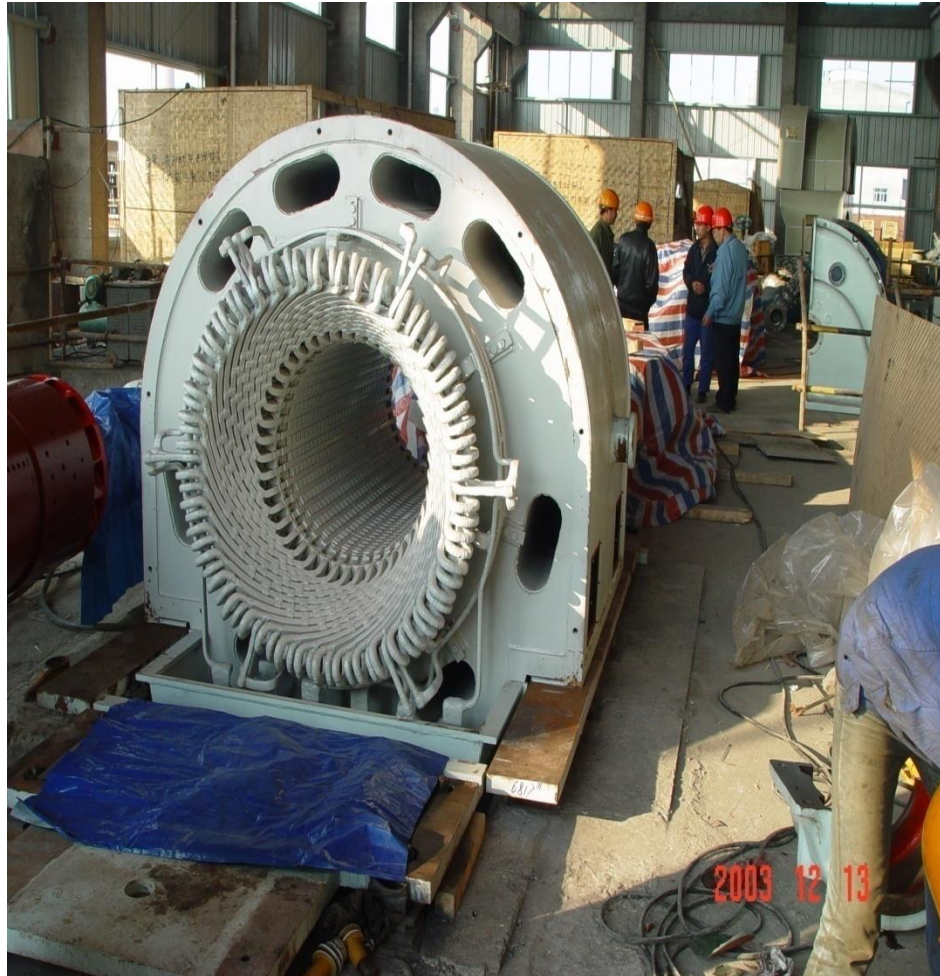
Install Stator and rotor generator unit
