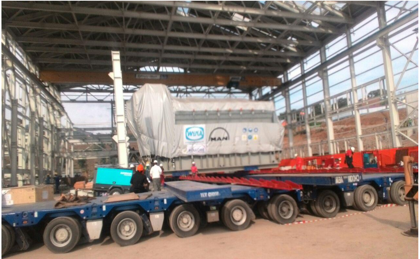
GAS ENGINE UNDER INSTALLATION ON FOUNDATION
