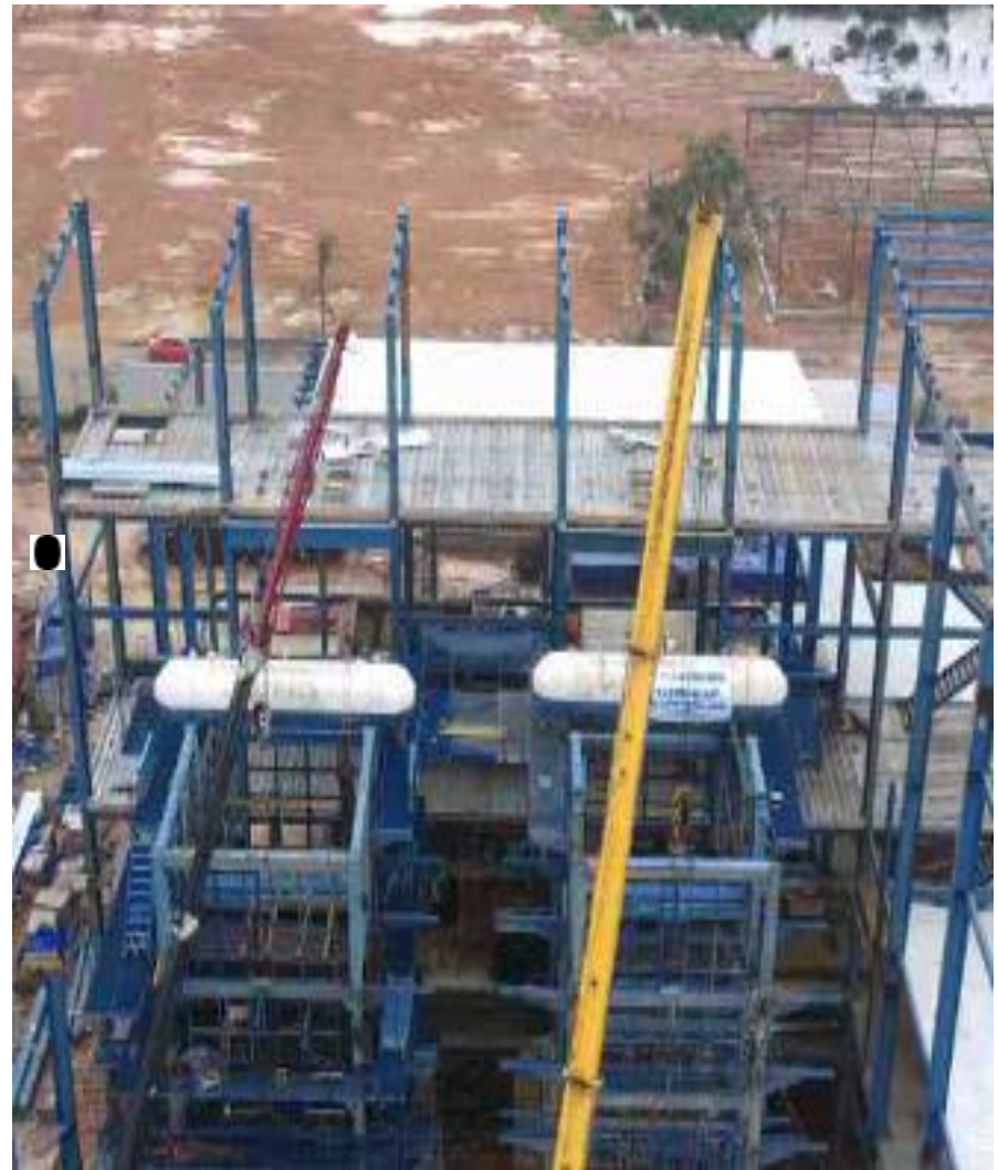
2 ( two ) unit steam drum fix at place)
