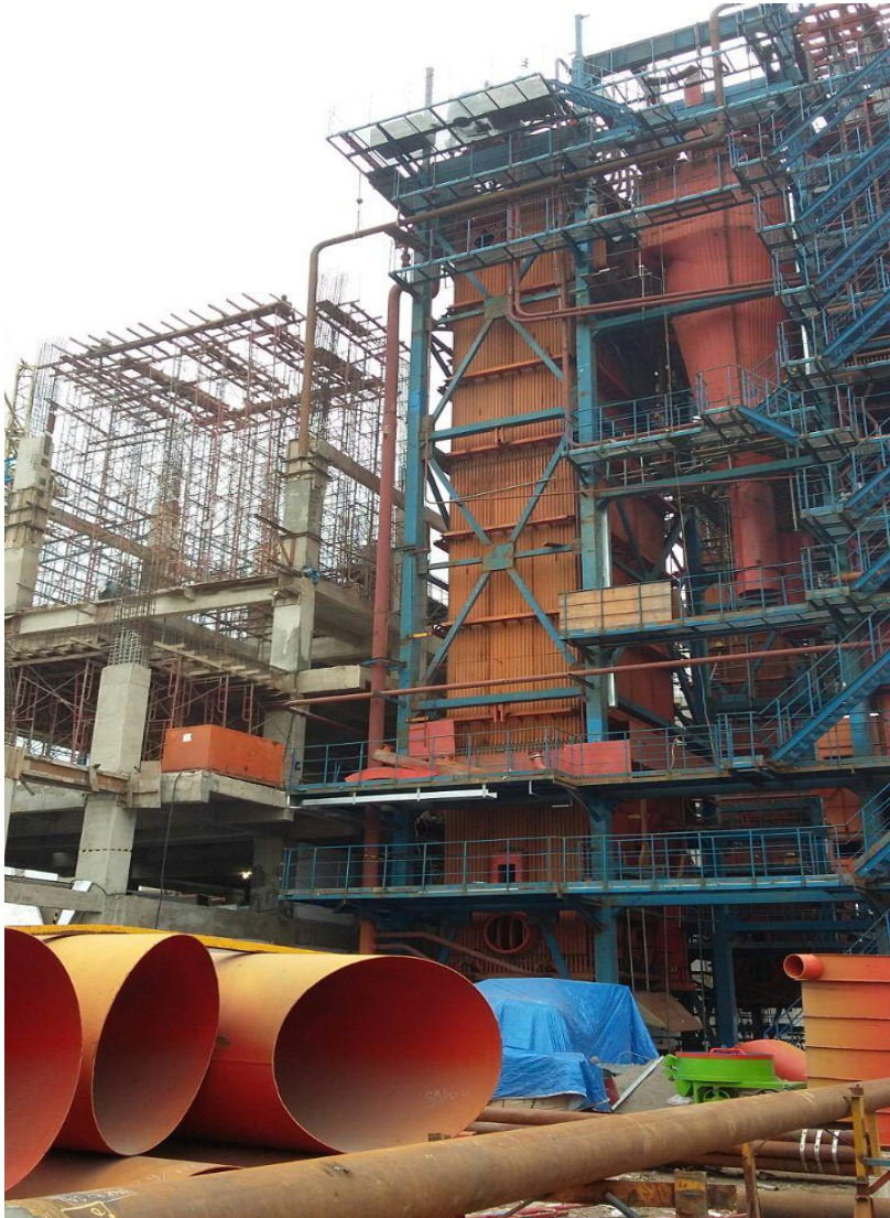
Install electrical / control cable
